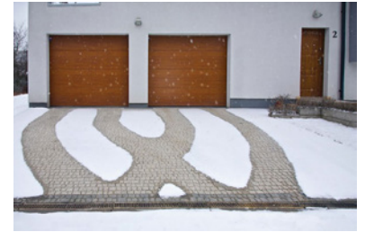
RESIDENTIAL DRIVEWAY SNOW MELTING
